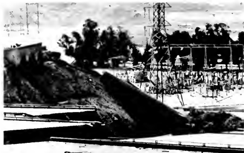
Photo 10. Damaged overcrossing at the Golden State Freeway and Foothill Freeway interchange [4].
